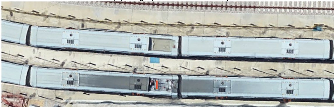
Figure 62 Photograph of roofs of two London Overground Class 378 electric multiple units, visually highlighting the effect of graphite and copper mixture lost from the pantograph wear strip (dark grey areas on lower train)
