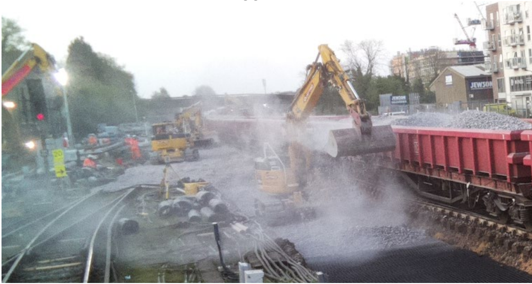
handling granite ballast
